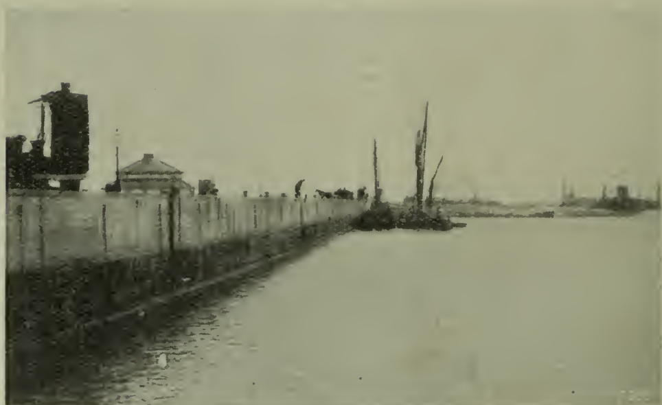
FIGS. 6 AND 7. TWO VIEWS SHOWING THE FINISHED QUAY WALL.
